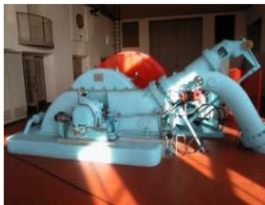
Figure 12: Mülhau: Drinking water turbine (2-nozzle Pelton turbine), from a micro hydropower installation that is part of a drinking water network.
