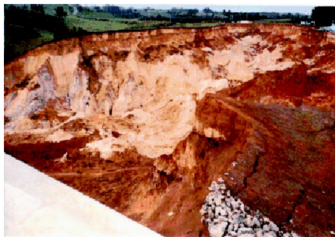
Figure 6: A photograph showing the effects of the Ruahihi canal failure.
